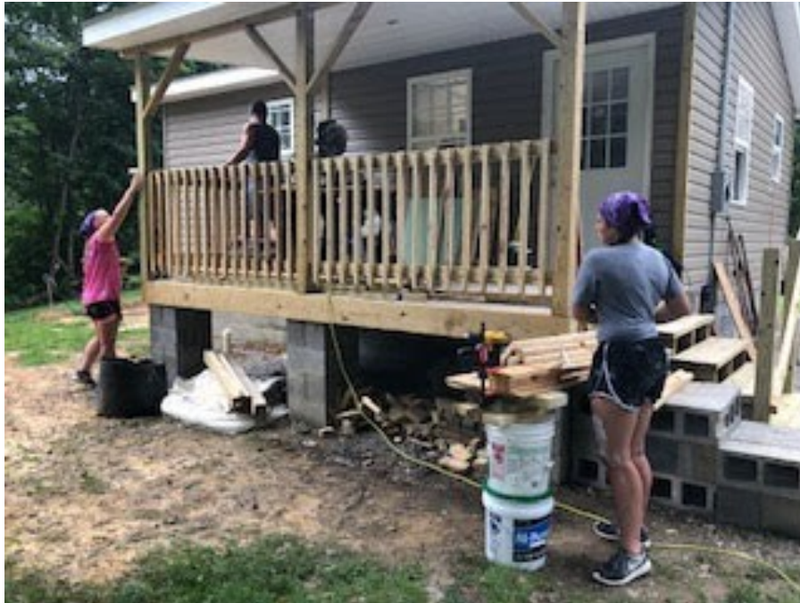
Nearing completion of Tom's new home. He has since moved in.
